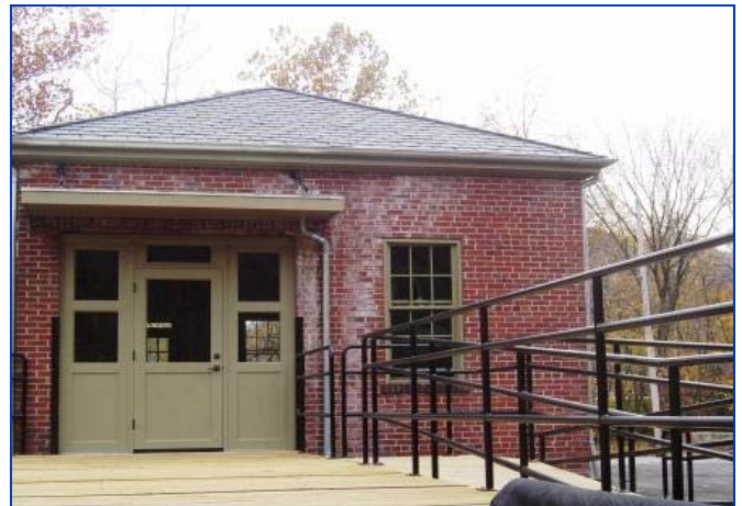
Spring 2011 View of Former Rail Depot Building Shows off the New Roof, Windows, Doors, and Exterior Additions
